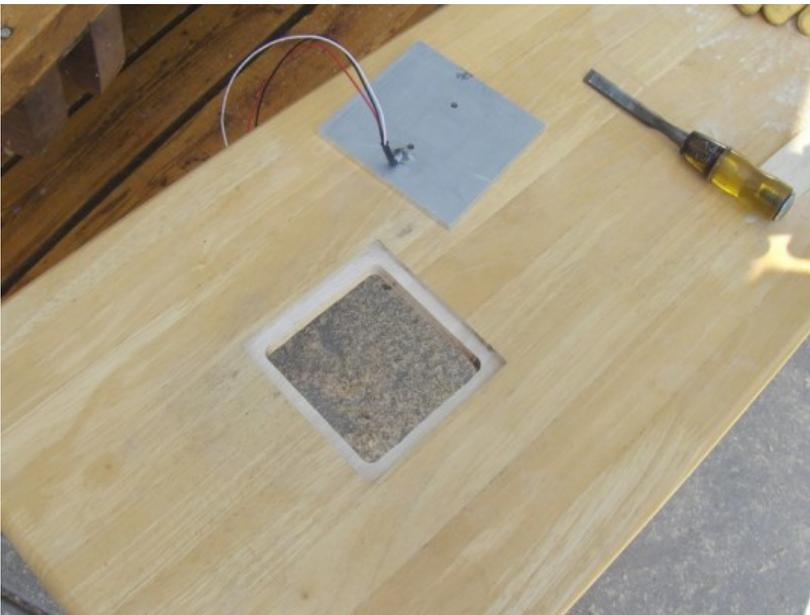
Using a router make an inset portion for the thickness of the surface plate. Then chisel out the corners.
